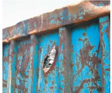
Scrap. A container made of a "mild steel" has cracked due to its poor resistance to wear, dents and blows. Not an attractive sight.
